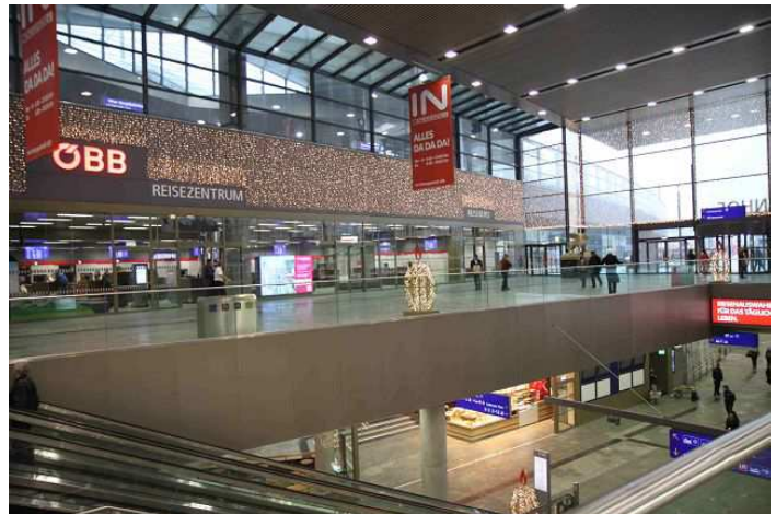
Vienna main railway station. Especially in the big waiting halls and in the main hall lighting lifts are used for the maintenance of lighting fixture
