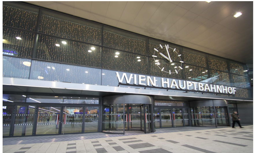
Vienna – Main railway station. Not everything that railway customers see is temporary Christmas decoration, but will be exchanged quickly and safely during the year without ladders or scaffolds using lighting lifts by REEL TECH.
