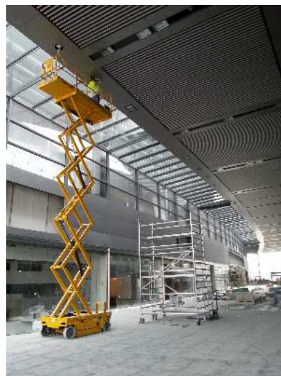
No longer necessary: heavy lifting platform for maintenance of lights at the high altitudes of the halls of Vienna Central Station
